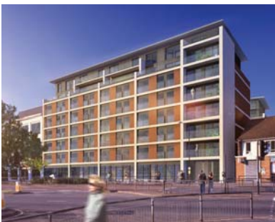
Mosaic Apartments, Slough
